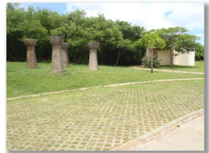
Photo 1: Permeable parking area at the Grotto, Saipan.
